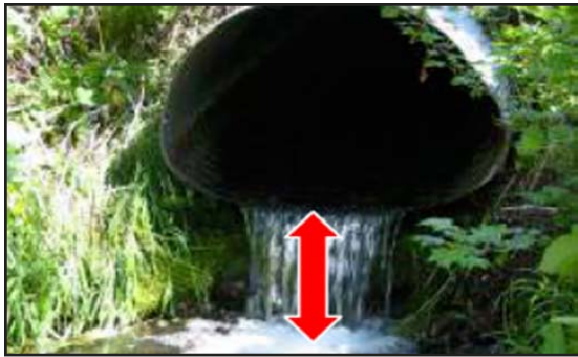
Photo (left): Perched culvert which is not fish friendly
