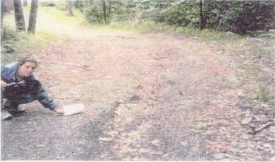
Photo 6- unstable culvert
